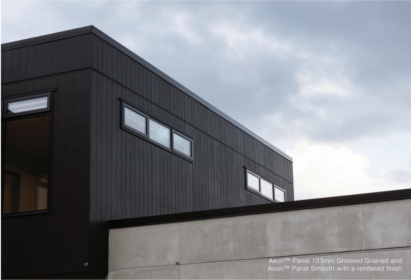
Axon™ Panel 133mm Grooved Grained and Axon™ Panel Smooth with a rendered finish
