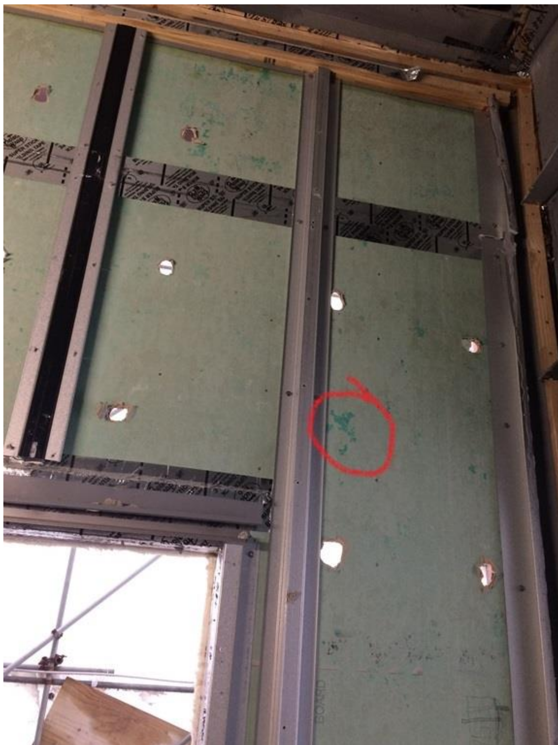
Figure 17: View from wet side of RAB board after removal of cladding, showing holes made in RAB board, and the damp patch from water seeping through the crack emanating from the head flashing.
