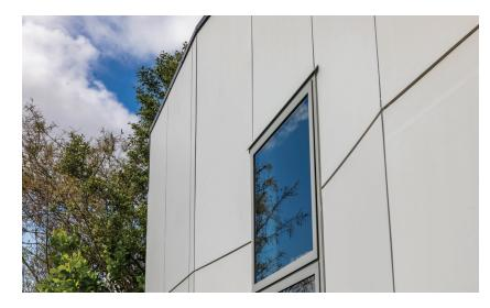
ExoTec<sup>™</sup> Facade Panel was applied across the exterior of the Marae building, replacing the aging metal cladding. This choice ensured the building retained its bold, modern appearance while benefiting from a contemporary, lowmaintenance solution.
